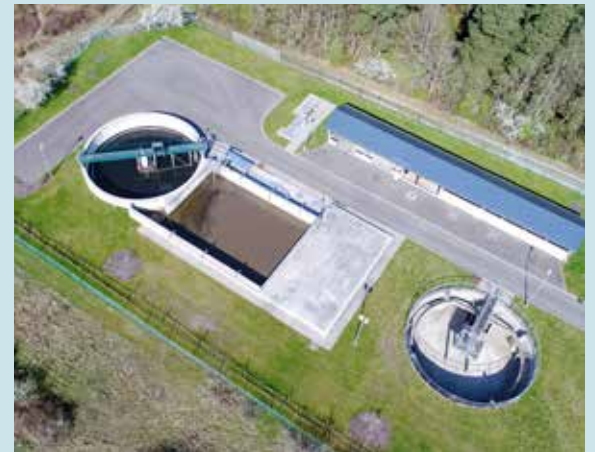
WASMUEL WASTEWATER TREATMENT PLANT | Belgium
