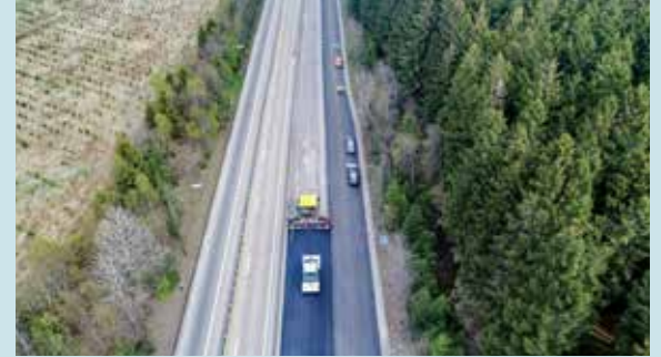
N4: trunk road Renewal of asphalt layer | Bastogne, Belgium
